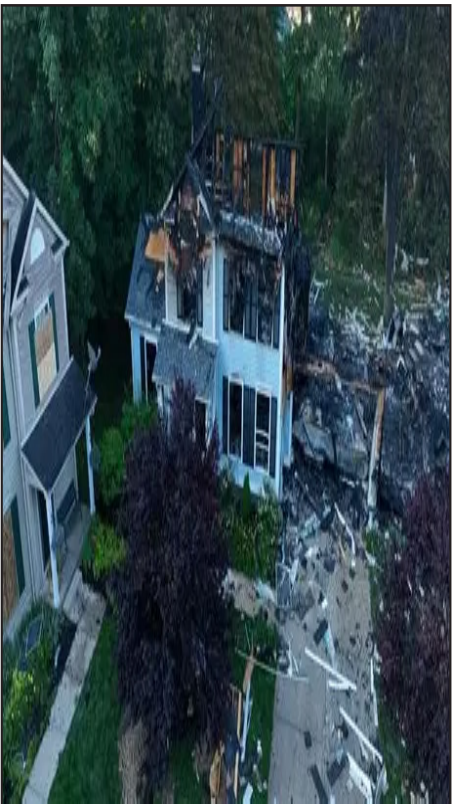
Homes in Twinsburg exploded. The incident occurred on Hiram Lane in the Woodlands neighborhood when contractors from Windstream’s Kinetic Fiber Internet team were working near a gas line
