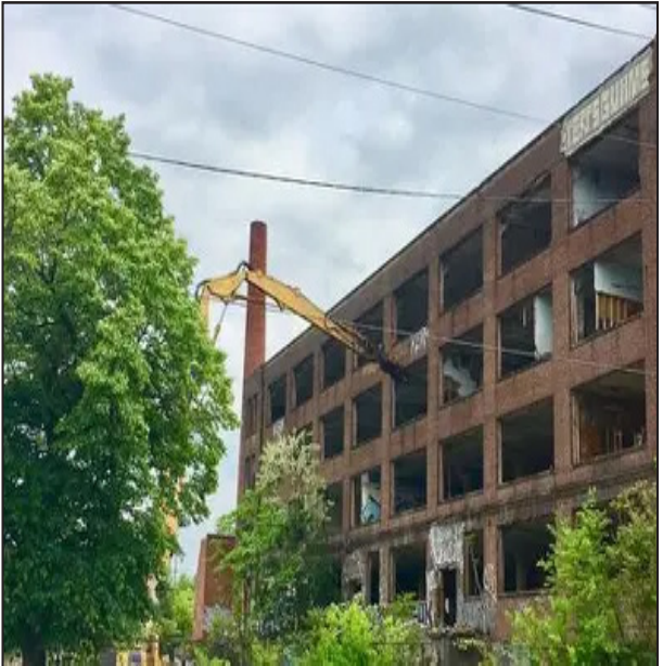
The Victoreen building, which has plagued Woodland Avenue for years was torn down in 2019. Cleveland Neighborhood Progress’s real estate arm was given the property for development. They have recently sold the property to the Industrial Landbank for $200,000,00
