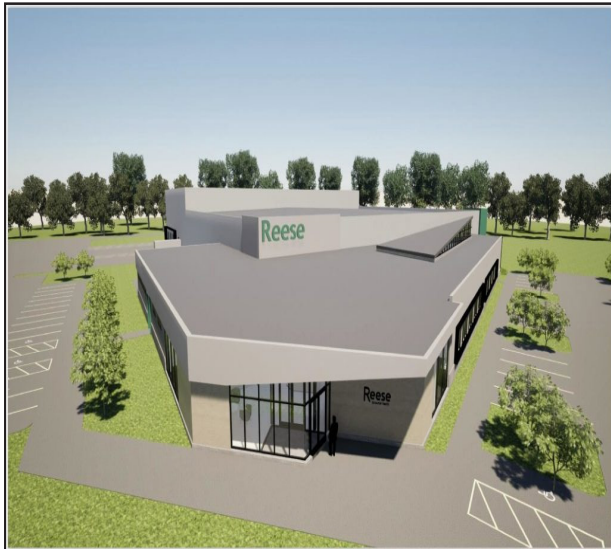
A new office building and production facility on Woodland Avenue near the Opportunity Corridor Boulevard for Reese Consumer Health was planned to allow the company to take advantage of growth opportunities. The project plans fell through and the company is looking to build in Slavic Village
